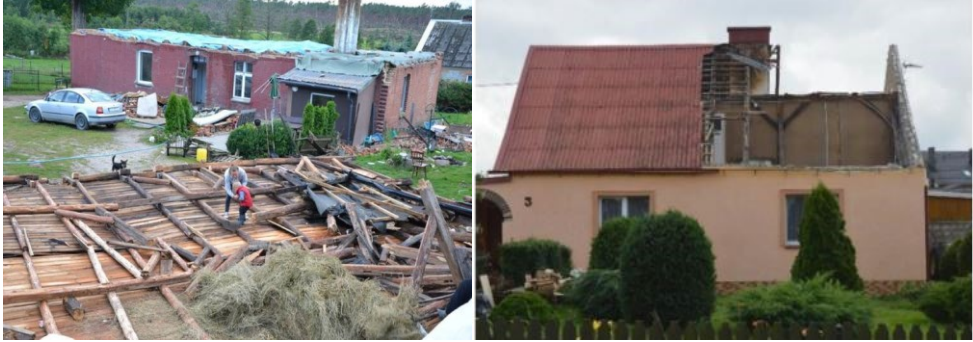
Fig. 5. Damage to buildings: entire roof blew off and part roof blew off from residential building.
