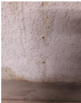
Fig. 3. Dampness in the connection between the diaphragm wall to the foundation slab.
