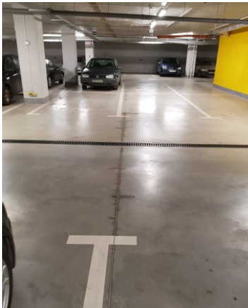
Fig. 1. Cracks in the parking slab with a width of over 0.6 mm.
