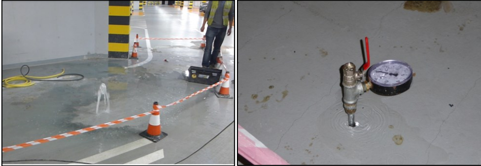
Fig. 2, 3. Drilling through the foundation slab and water pressure measurement.
