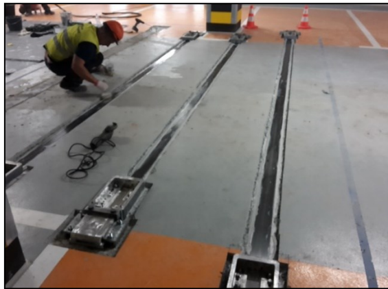
Fig. 9. View of the stripes after prestressing – preparation to reprofiling of finishing layer.
