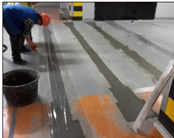
Fig. 10. View of the floor after reprofiling with PCC mortar.
