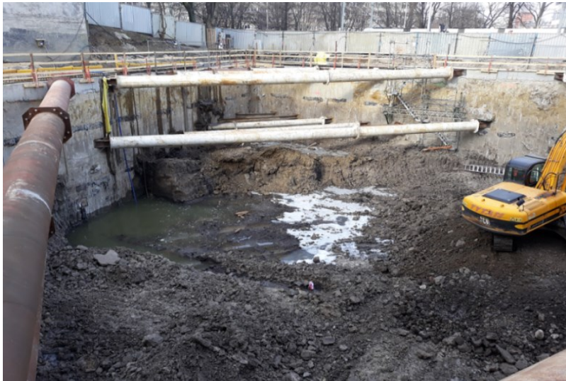
Fig. 4. Excavation works in progress.
