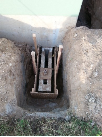
Fig. 13. Formwork for beams after rectification.
