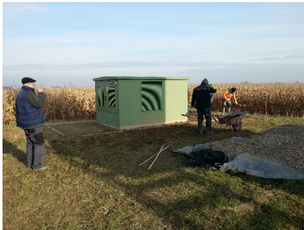
Fig. 15. Backfill after the repair.
