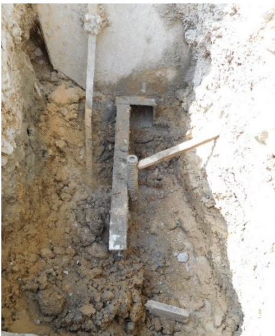
Fig. 7. Installation of steel beams 2xC140.
