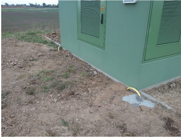
Fig. 16. Injection used to fill any voids under the plate.
