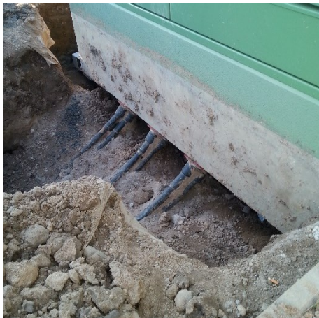
Fig. 11. Tightening power cables.
