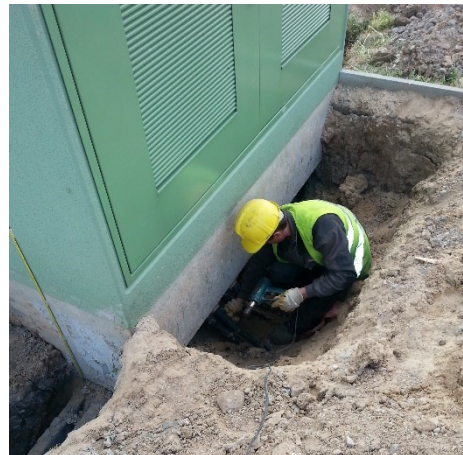
Fig. 12. Sealing cable entries after lifting.
