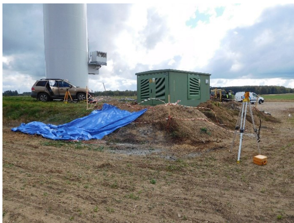
Fig. 9. Control of lifting using two levelling instruments.
