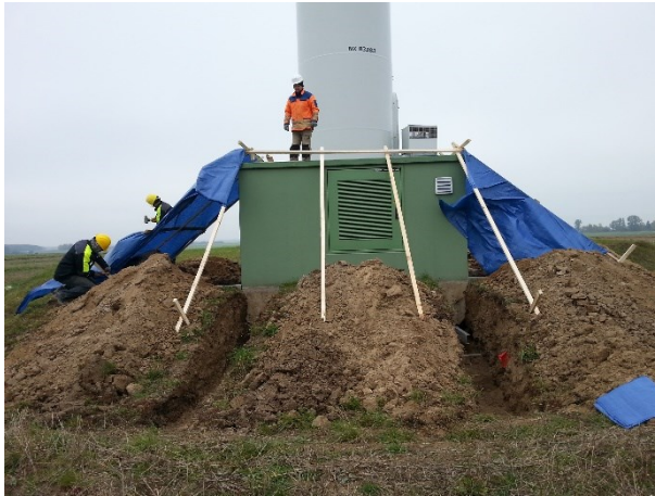
Fig. 5. Rainwater protection concerning the transformer station area.
