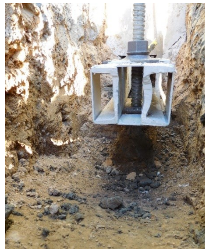
Fig. 8. Supporting support beams on micro-piles.
