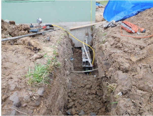
Fig. 10. Lifting the corner using a hydraulic cylinder and a manual pump.
