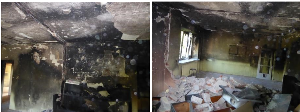
Fig. 6. The view of the destroyed partition wall between apartments no. 109 and 110.
