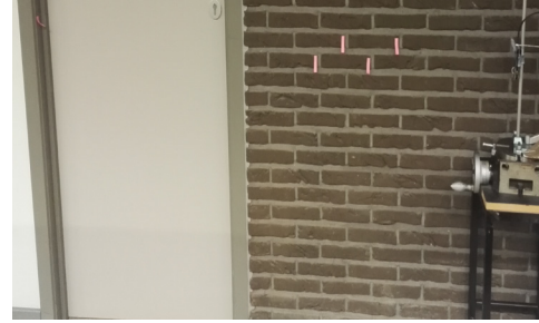
Fig. 5. Measurement of the wall.
