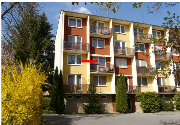
Fig. 1. Case study pre-cast concrete building – T 06 B – KD building system, view of markedly broken façade with protruding walls and balconies. Red mark points to the place of the cross section in the assessed critical detail.
