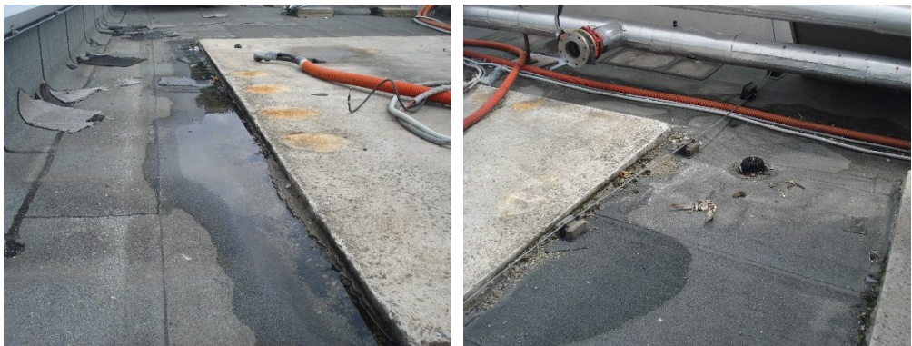
Fig. 1, 2. Pushing of distributing concrete structure to roof cladding
