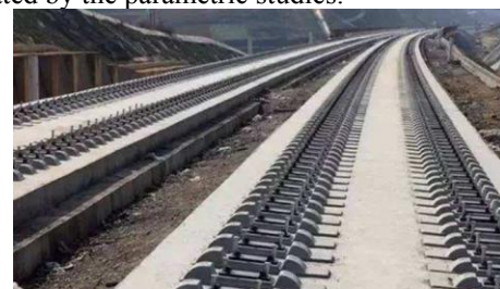
Fig. 1. Adjacent railway tracks in track engineering
