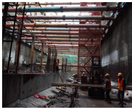
Fig. 6. Row pile and inner support structure.
