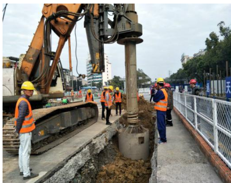
Fig. 5. Rotary drilling rig construction.
