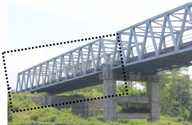
Fig. 1. The approach bridge of Kalimujur Bridges.
