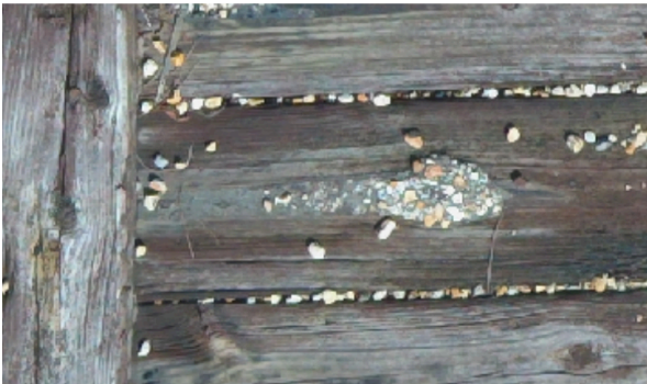
Fig. 5. Zoom view of bridge deck.
