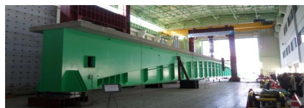
Fig. 9. SBarch fabrication process at workshop
