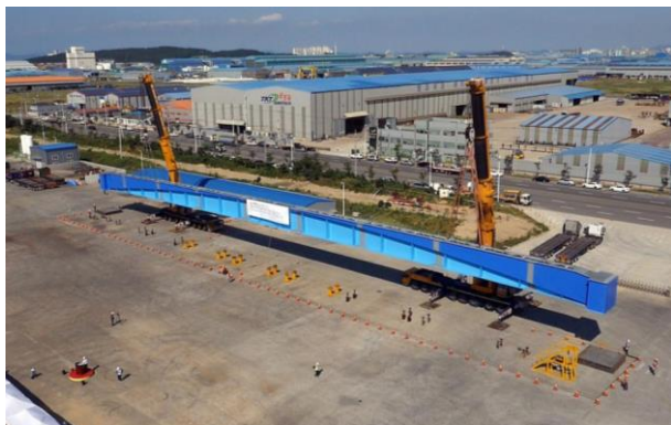
Fig. 10. Sbarch erection process using crane lift
