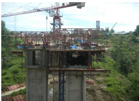
Fig. 1. Cast in-situ balanced cantilever
