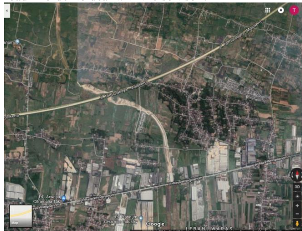
Fig. 12. The construction of Krian Legundi Bunder Manyar Toll
