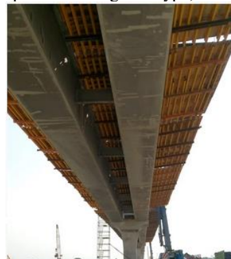
Fig. 3. Steel box girder
