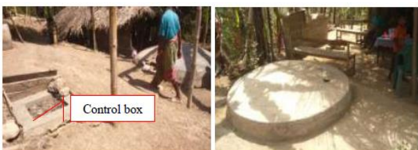
Fig. 10. Control box from mineralization process for clean water tank
