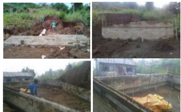
Fig. 12. The construction of reservoir below the home-stay for tourism
