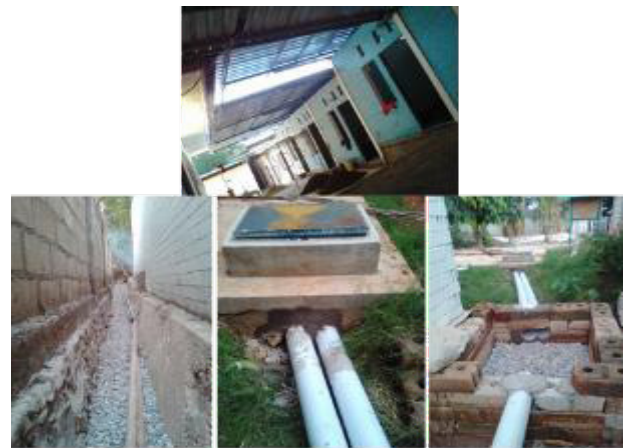
Fig. 11. Rainwater management construction in Nasipanaf, Kupang Regency dormitory
