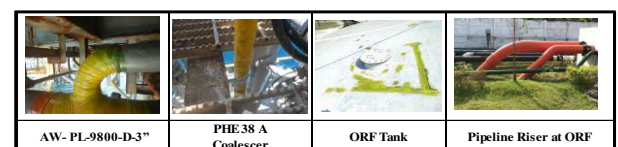
Fig. 3. Inspection Activity and Picture of Composite Repair Visual
