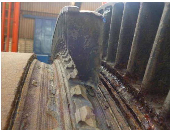
Fig. 5. Heavy corrosion damage in the loading slots of the rotor.
