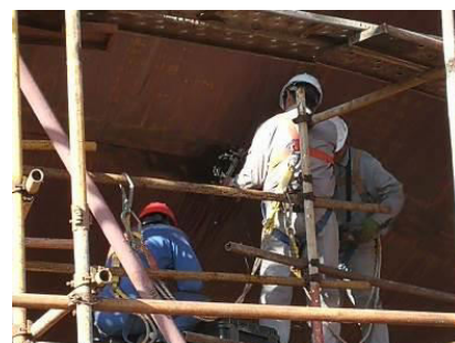
Fig. 2. Manual weld inspection of spherical tank.
