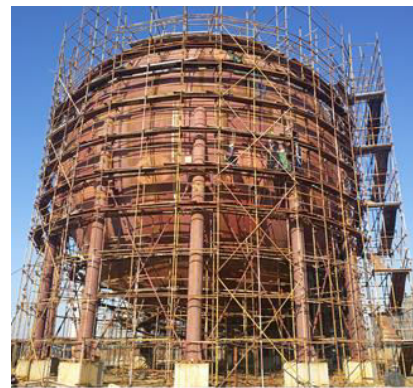
Fig. 1. Spherical tank in the construction.
