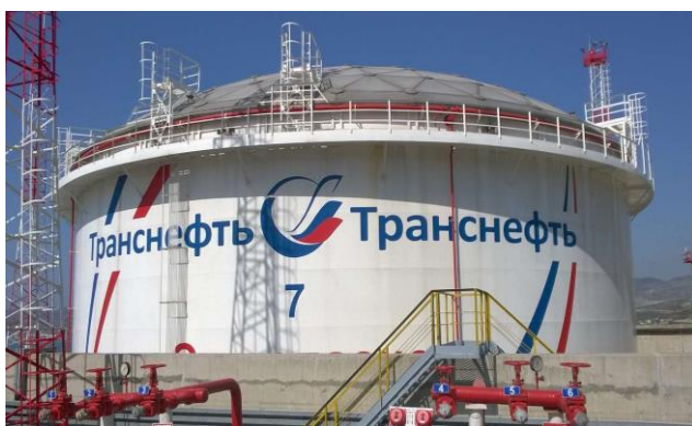
Fig. 1. Vertical cylindrical steel oil storage tank.
