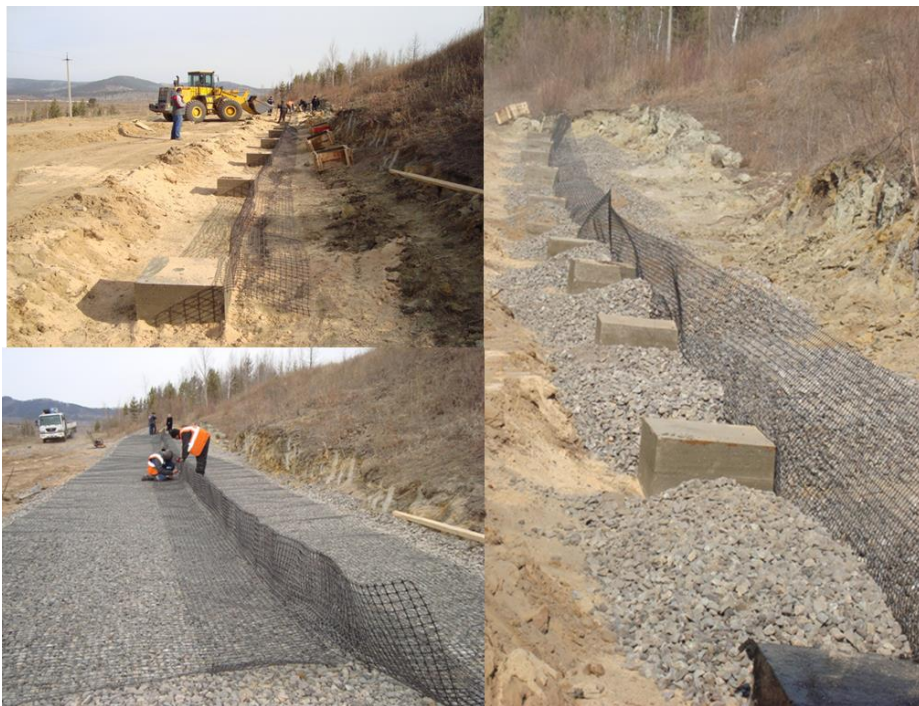
Fig. 7. Pile caps installation, crushed stone filling, geogrid fastening with binding.
