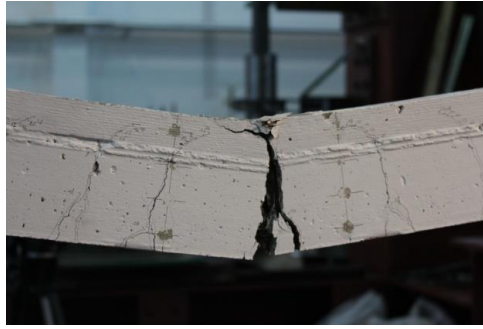
Fig. 3. Failure of beam due to concrete crushing.
