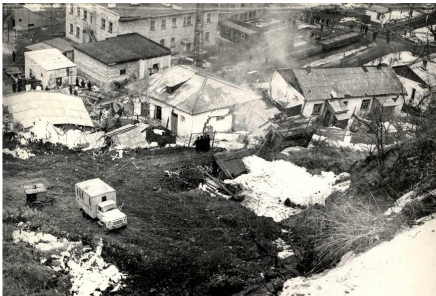
Fig. 3. The Nevelsk Town, may 1981. Landslide destroyed 5 residential houses. The West coast of Sakhalin Island.
