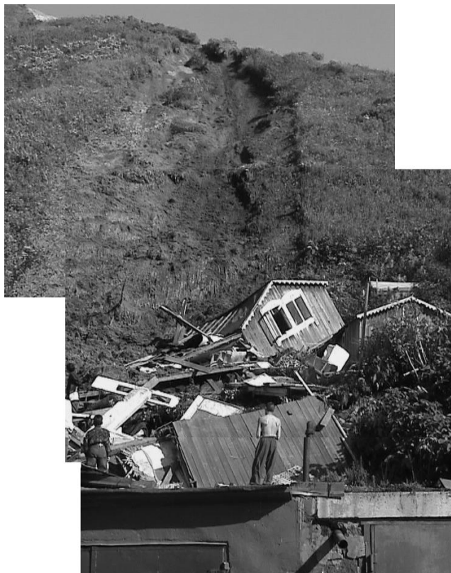
Fig. 4. Residential house destroyed by a landslide.
