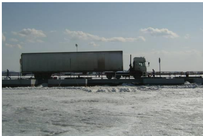
Fig. 2. Configuration of the loaded vehicle passage with the "threshold" and in the span.
