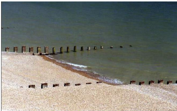
Fig. 7. Concrete groyne structures protection.
