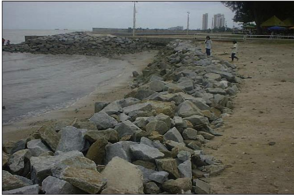
Fig. 6. Rock revetment used for erosion.
