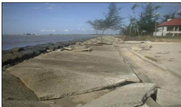
Fig. 5. Concrete units used for erosion protection.
