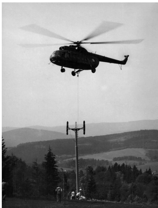
Fig. 1. Erection of pipe supports of the Špičák - Pancíř chairlift ropeway.
