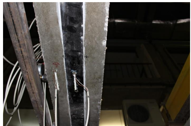
Fig. 5. CFRP strip on the bottom surface of RC beam.
