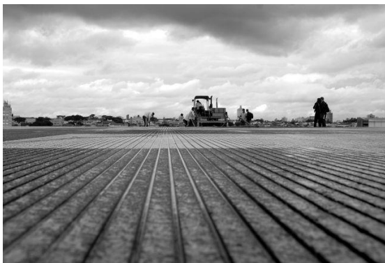
Fig. 1. An example of a grooved airfield pavement in the cement concrete technology [source: www.nasa.gov ].
