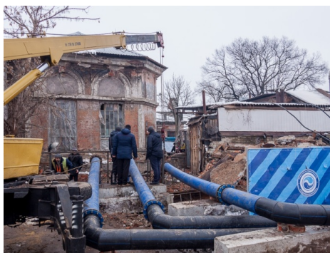
Fig. 1. Temporary disposal of wastewater.
