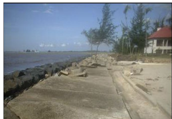
Fig. 11 Concrete units used for erosion protection
