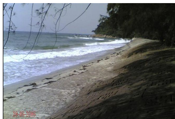
Fig. 16 The condition of shoreline before application geotextile tube protection works (June 2006)
