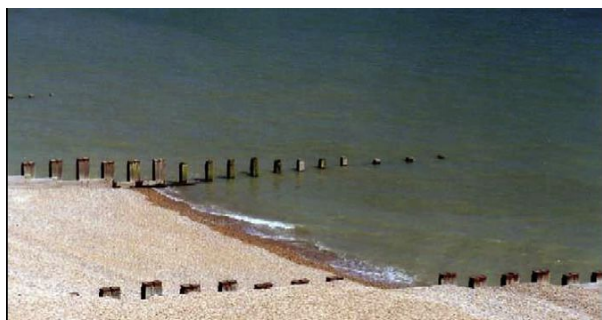
Fig. 13 Concrete groyne structures protection
