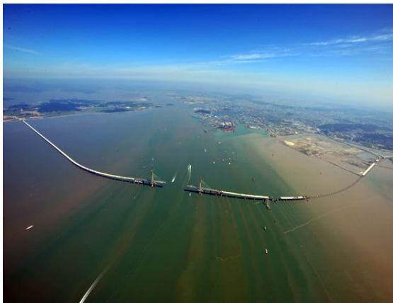
Fig. 1 Incheon Bridge linking IIA and IFEZ in 2010
