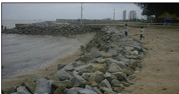
Fig. 12 Rock revetment used for erosion
