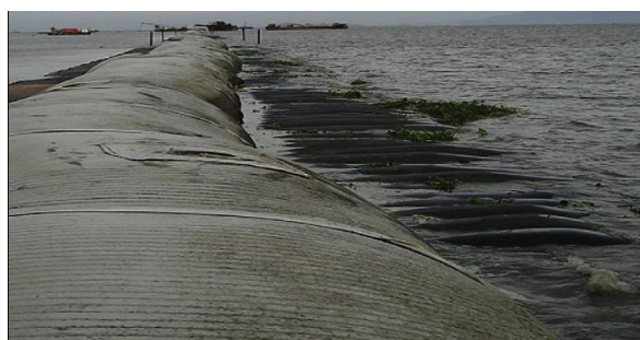
Fig. 15 Geotextile tube used for coastal protection works
