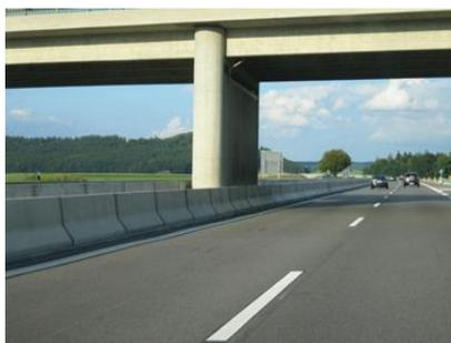
Fig. 1. Concrete barrier protecting the bridge column (source: [www.debonte.com](http://www.debonte.com)).
