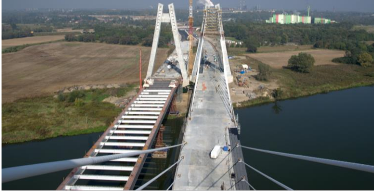
Fig. 1. The bridge MD-7 under construction.
