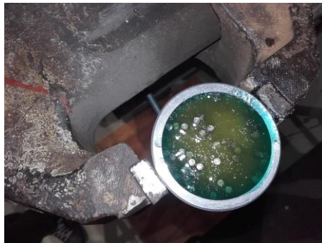
Fig. 6. WIRELOCK resin after the curing process.
