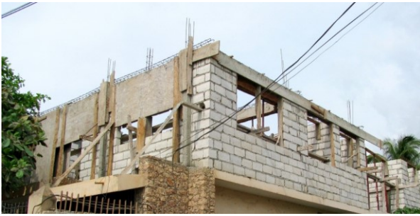
Figure 5 Confined masonry: formwork present after construction of walls; note lack of columns on right side. [30]
