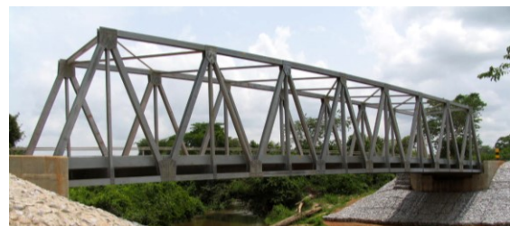
Figure 1 Truss Steel bridge [5].
