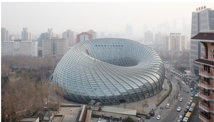
Fig. 3. The International Media Center "Phoenix" in Beijing (Chao Weiping). The idea of the Mobius strip is embodied by the parametric modification of the cells of the shell of a building.
