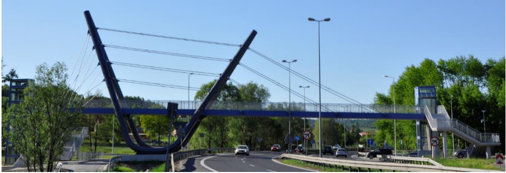
Fig. 1. Side view of the cable-stayed footbridge.
