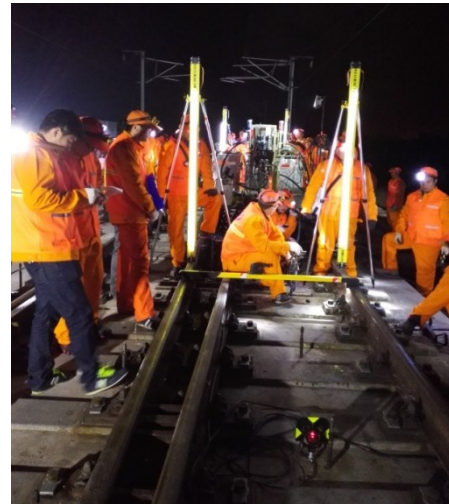
Fig. 4. Polymer injection rehabilitation for lifting differential settlement of turnout ballastless track
