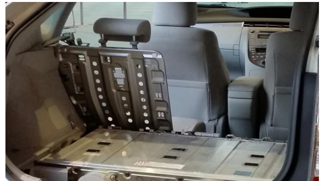
Figure 1. Ni-MH battery packs in a hybrid vehicle.
