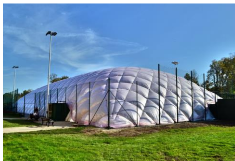
Fig. 3. Three-layer pneumatic hall with a protective mesh made of steel cables; source: [20]
