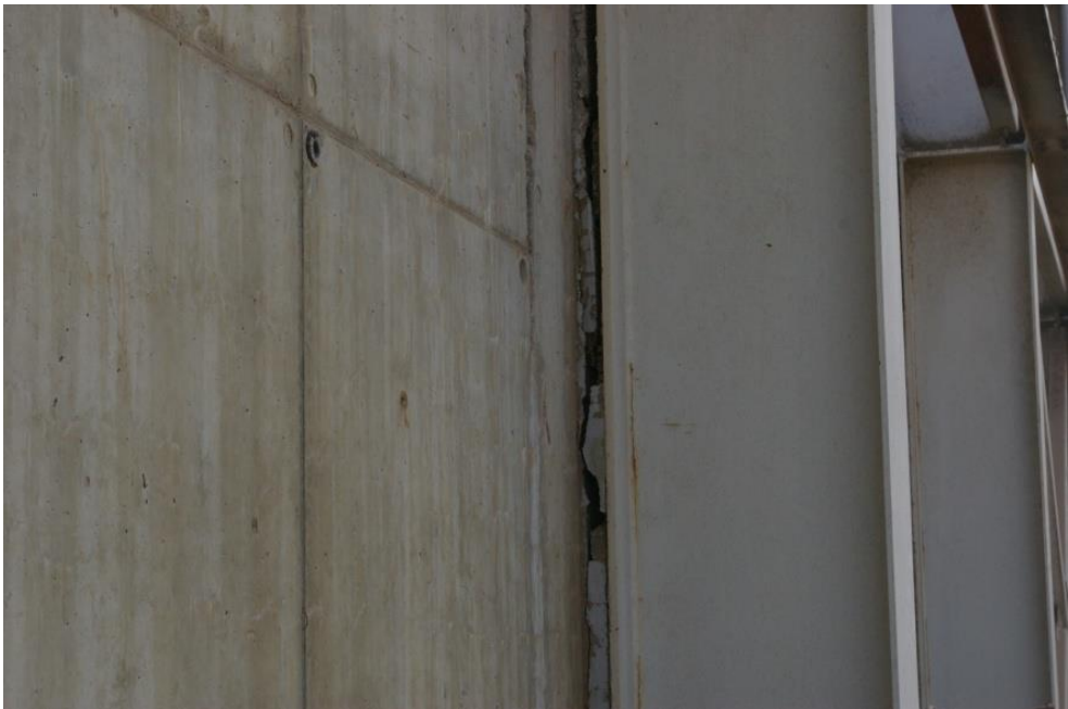
Fig. 6. Bottom part of the column in the axis C-14 .
