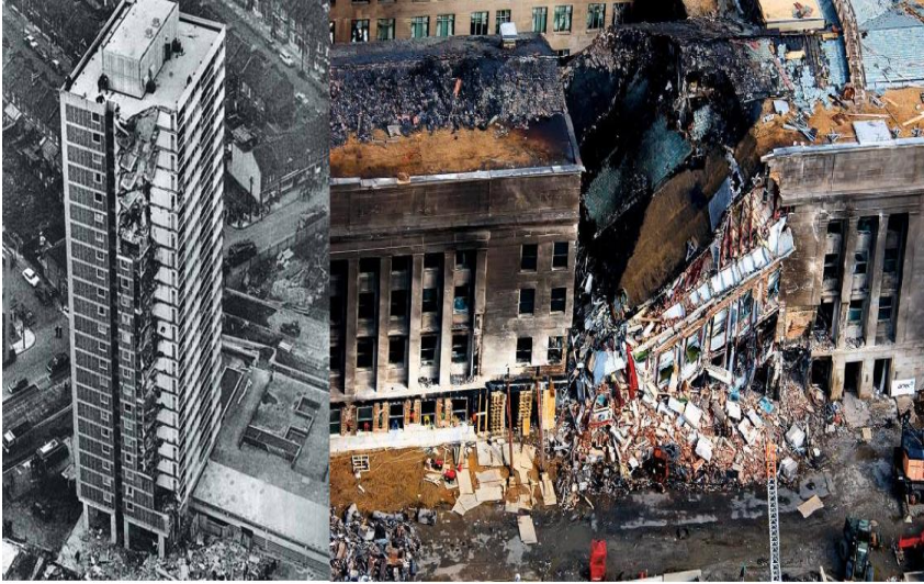
Fig. 1. Progressive collapse of buildings
