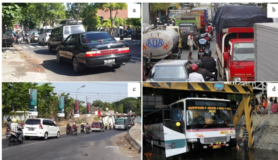
Fig. 1. Problems of the existing Gilingan Viaduct.
