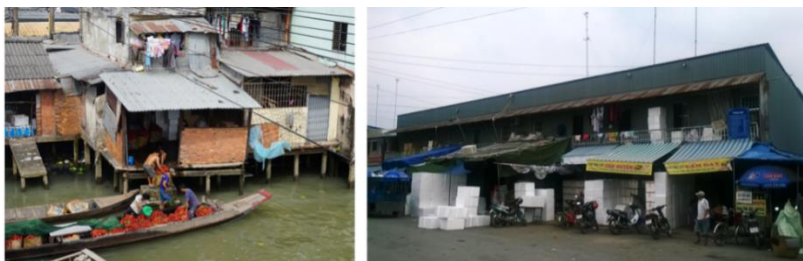
Houses on stilts in Mekong delta with the front face water (left) and face road (right)
