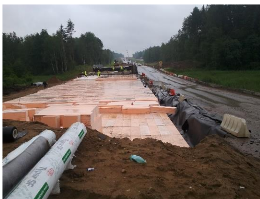
Fig. 1. The erection of a light embankment on a weak base
