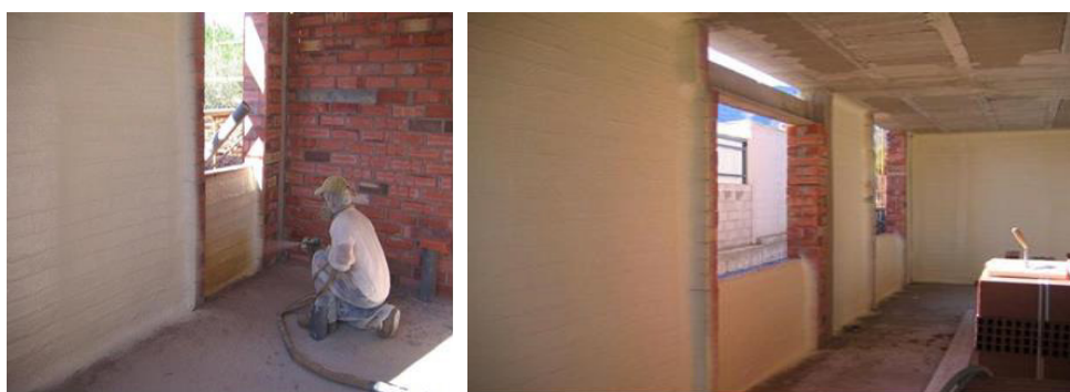
Fig. 1 - Application of polyurethane foam for thermal insulation
