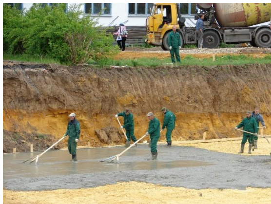
Fig. 1. Fragment of the soil profile in the building pit in the Nizhny Novgorod region of Russia.
