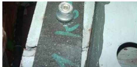
Fig. 12 Repair of hinge console
