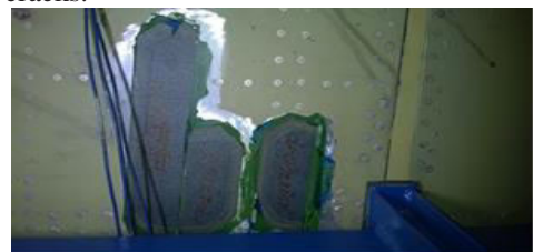
Fig. 14 Repair by composite patches
