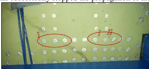
Fig. 13 Cracks on wing skin to be repaired
