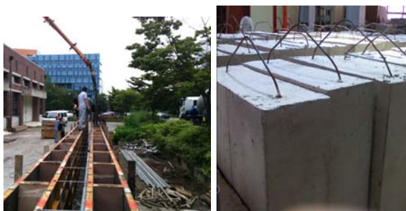
(a). Construction of concrete specimen
