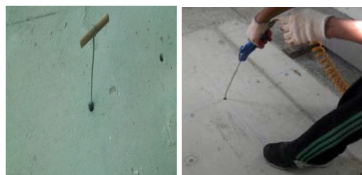
(c). Clean up for anchor installation
