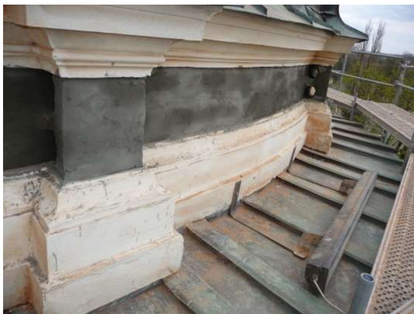
Fig. 7. The preparation of the church dome's drum for placing CFRP strips.
