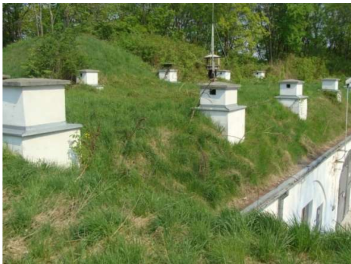
Fig. 7. Roofing of the building facility No. 60.
