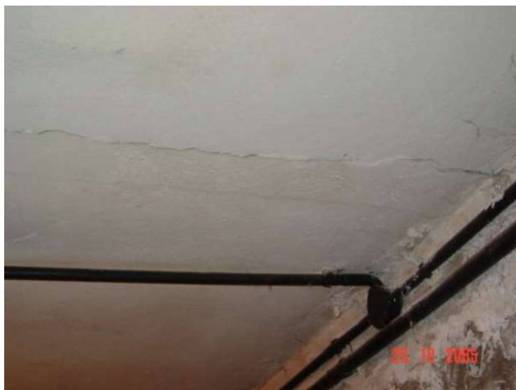
Fig. 2. Ceiling above the basement of the eastern outbuilding.
